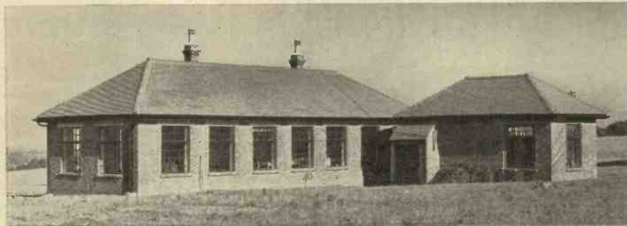
The Tatsfield station consists of two buildings. The one on the right is the power house and that on the left houses the checking apparatus.
